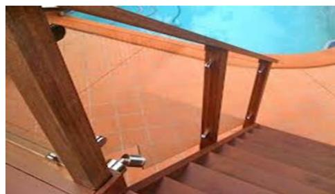
2) As a Structural Balustrade Panel (Figures 1 & 2) where the glass is the main structural component of the balustrade.
