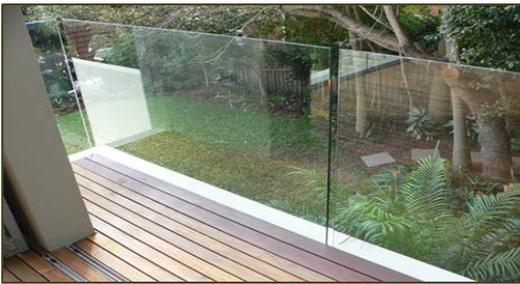
**Figure 5 - Structural Balustrade A: Non-compliant above 1 metre fall height. (Source: [www.elitebalustrades.com.au](http://www.elitebalustrades.com.au))**
