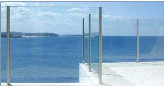
**Figure 6 - Structural Balustrade B: Non-compliant above 1 metre fall height. (Source: [www.eglasame.com](http://www.eglasame.com))**
